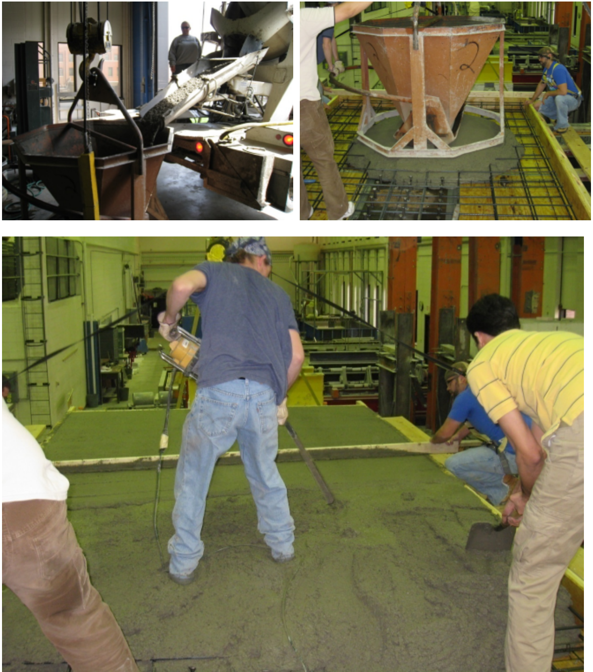
FIGURE 2-9: CONCRETE POURING PROCESS
