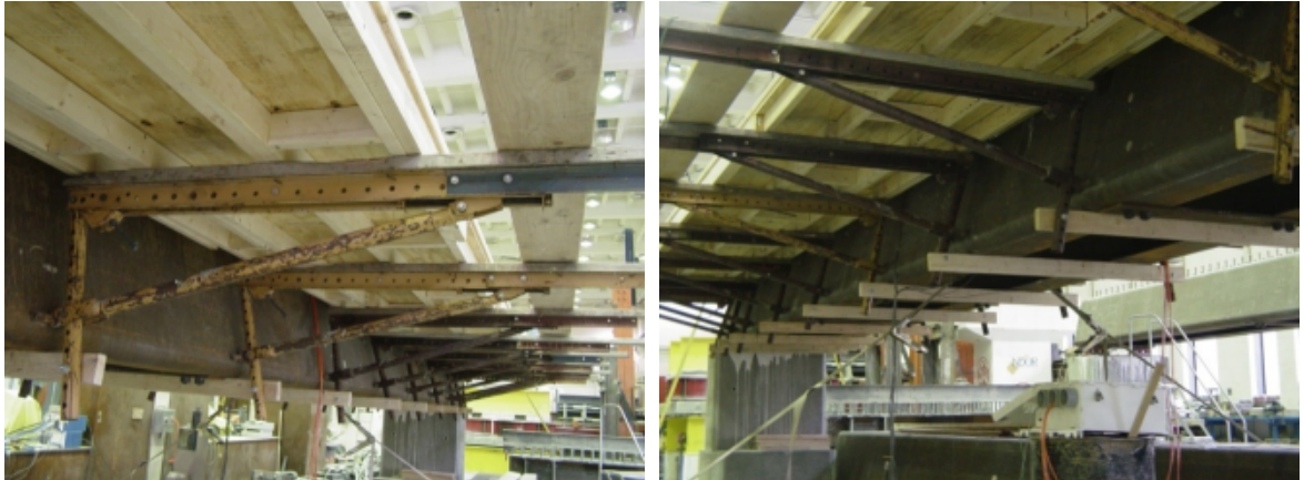
FIGURE 2-6: KNEE BRACES USED TO SUPPORT WET CONCRETE
