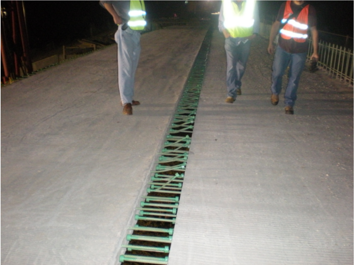
FIGURE 5-1: HEADED REBAR IN LONGITUDINAL JOINT
